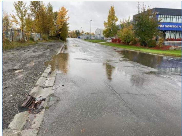
Widespread ponding & ineffective catch basin at the Quinhagak Street and E. 64 th Avenue intersection
