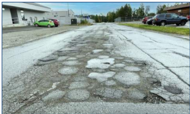
Poor roadway conditions along Quinhagak Street require regular attention from MOA Street Maintenance
