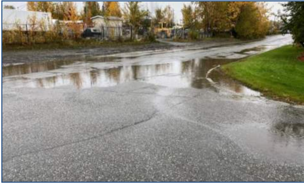
Flat grades & heaved curbs result in ponding at the Quinhagak Street & E. 63 rd Avenue intersection
