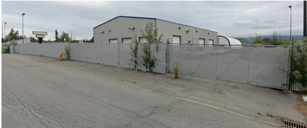
Photo 1 – Parcel 3 Driveway Gate Fence with Slats
